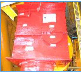
Completed 36" Main SDV, installed and fitted with its PFP castings and wet applied PFP.
