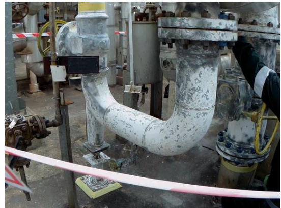
Mechanical preparation to ST2
