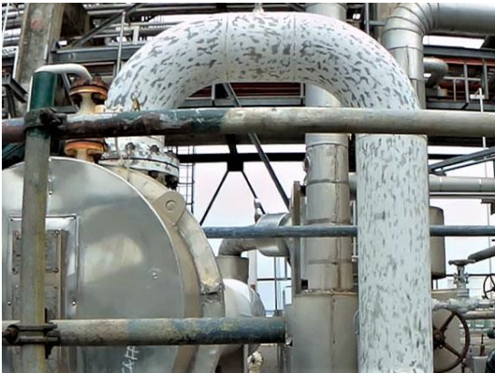
Mechanical preparation to ST2
