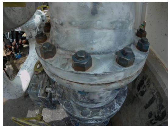
Mechanical preparation to ST2
