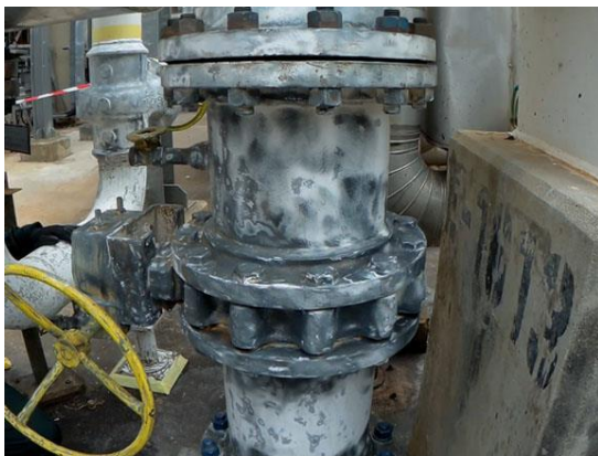
Mechanical preparation to ST2
