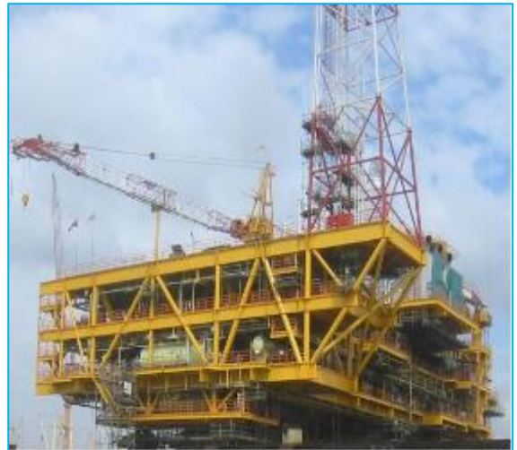
HELANG TOPSIDES PROJECT
