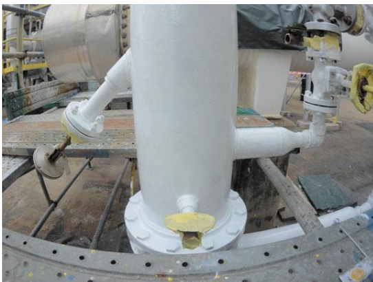
Coating applied during hot surface temperature
