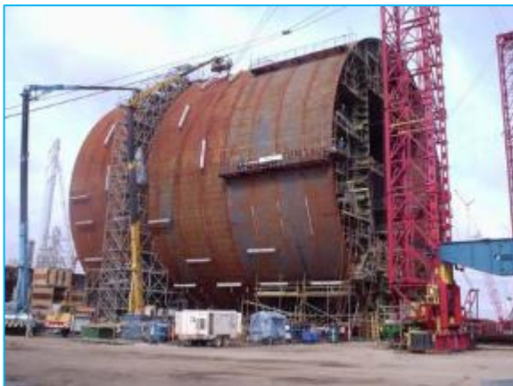
KIKEH DTU TRUSS SPAR PROJECT
