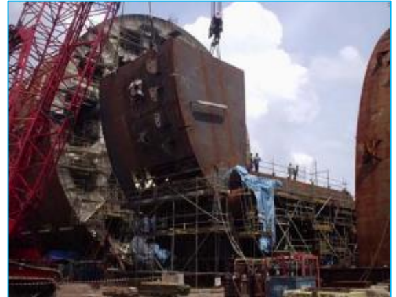
KIKEH DTU TRUSS SPAR PROJECT
