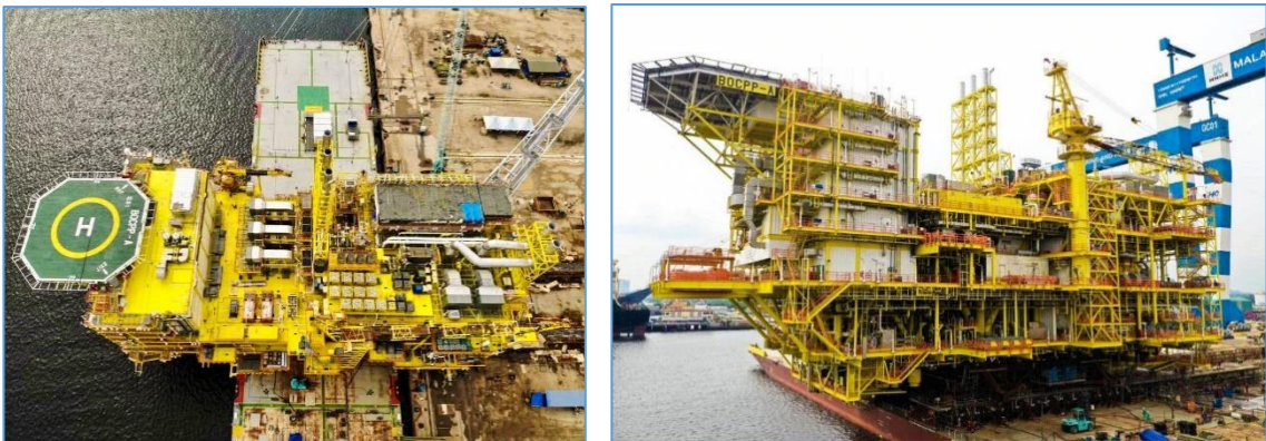
BOKOR CPP Project - Loadout and Sail away (Aug 2020)
