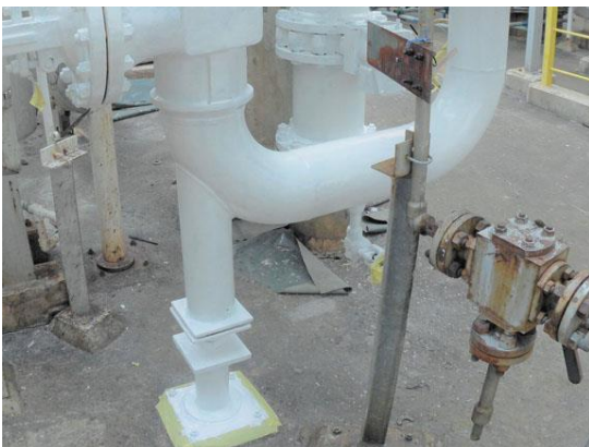
Coating applied during hot surface temperature
