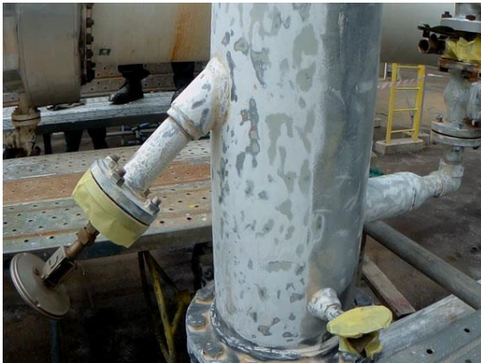
Mechanical preparation to ST2
