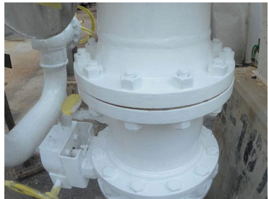
Coating applied during normal surface temperature
