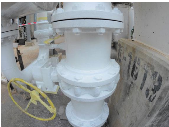
Coating applied during normal surface temperature
