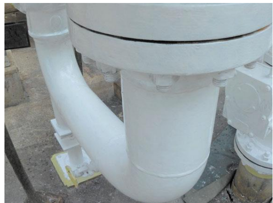
Coating applied during hot surface temperature
