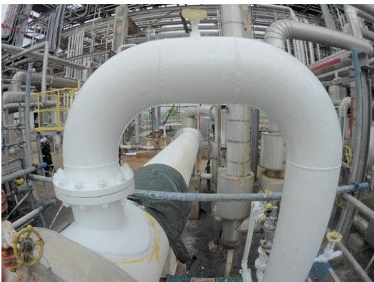
Coating applied during hot surface temperature
