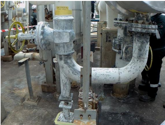
Mechanical preparation to ST2
